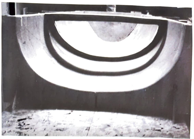
TB-2 and TB-3 installed.
